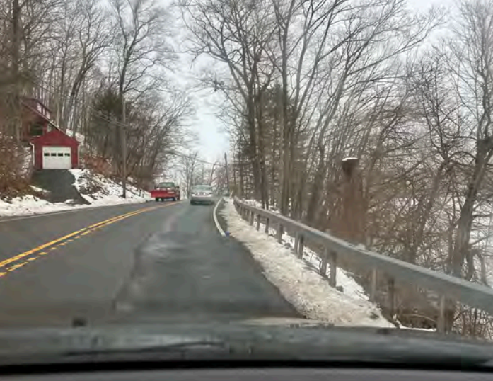
Box beam rail at Lake Quonnipaug in Guilford (VHB)
